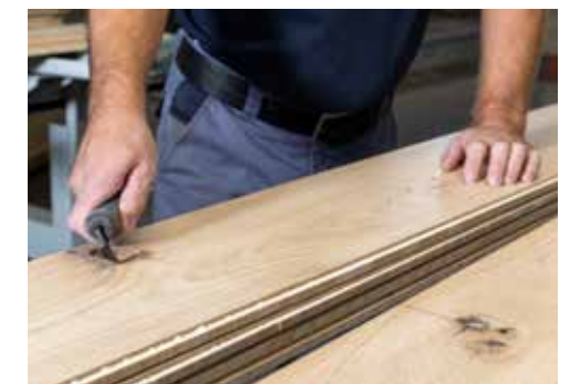
Scraping out of loose fibres before the puttying.
